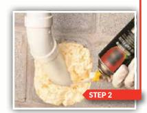
Step 2: Spray foam into steel wool.
