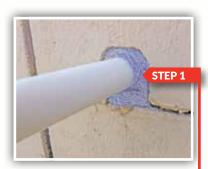
Step 1: Fill gap with coarse steel wool.
