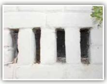
Check for loose mesh in foundation vents.
