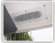
Soffit vent hole sealed with screen.\*
